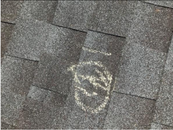
This picture shows torn shingle on back elevation
