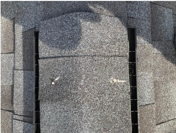
This picture shows sealant on exposed nail heads at peak of roof elevation
