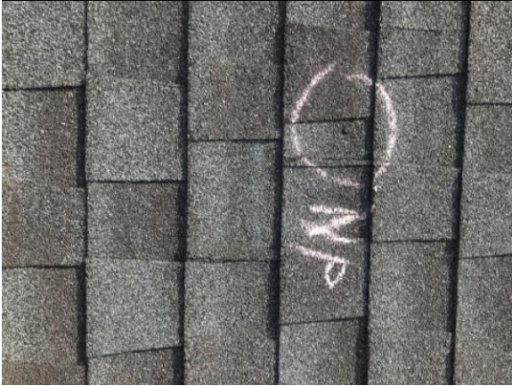
This picture shows nail popping through the shingle on back elevation
