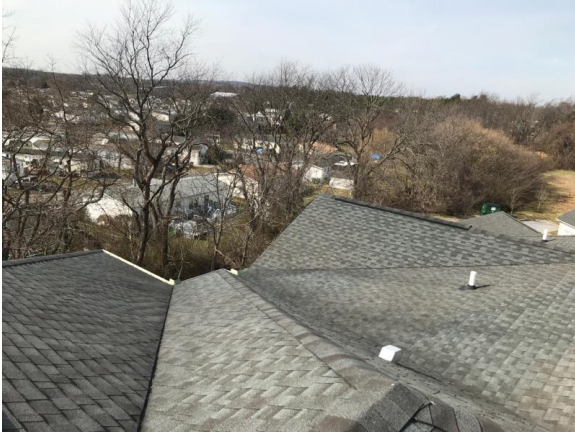
This picture shows over view of back elevation and some staining from algae growth
