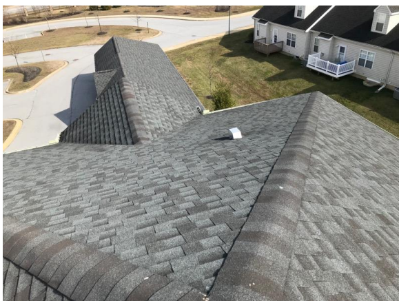
This picture shows hipped roof elevation and cap shingles
