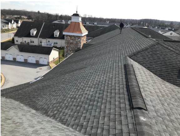
This picture shows overview of the middle elevation and the ridg vent system
