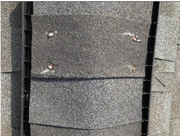
This picture shows exposed nail heads at peak of ridge vent. Sealant is recommended
