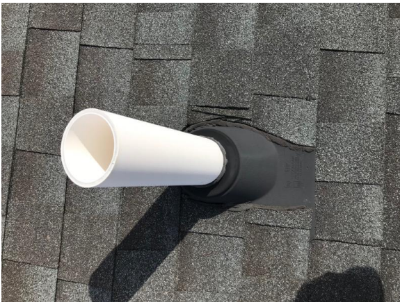
This picture shows pipe collars appear to be in good condition
