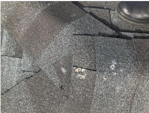
This picture shows some additional damage at peak of hipped roof that appears to be done by birds landing on this area
