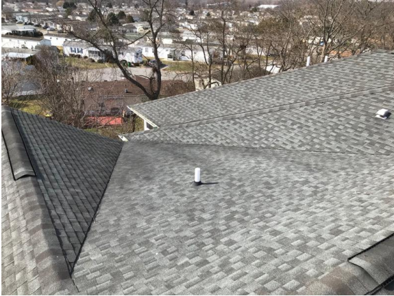
This picture shows gusset valley and some staining algae growth
