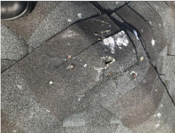
This picture shows some damaged shingle at peak of hipped roof. This maybe caused by birds landing on this spot. Replacement of these shingle are recommended
