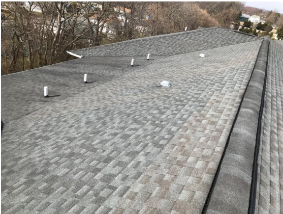
This picture shows pipe collars on back elevation appear to be in good condition
