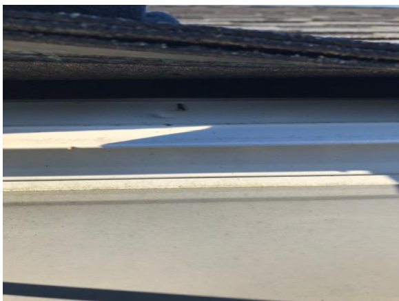
This picture shows there is drip edge on the roof and appears to be installed correctly
