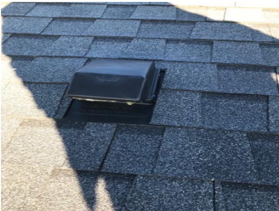
This picture shows bathroom and dry vents have some debris in them and cleaning is recommended.
