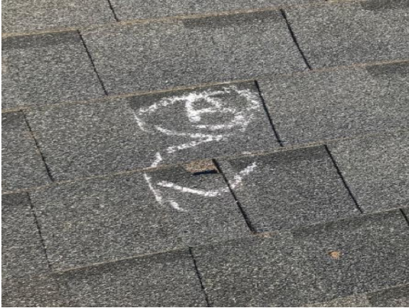
This picture shows additions damaged shingles on back elevation
