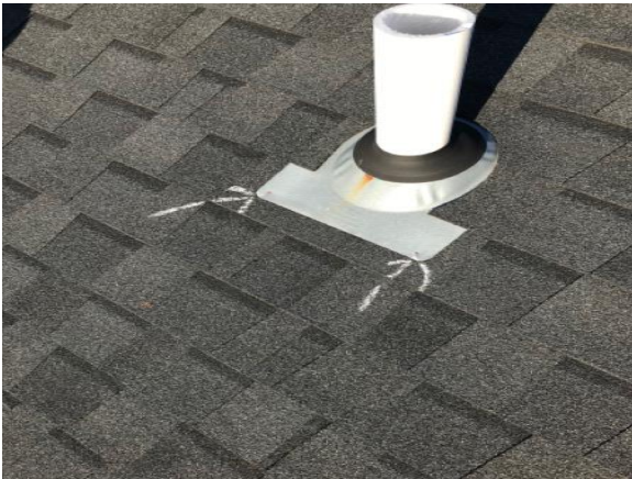
Tis picture shows exposed nail heads on pipe collars. Sealant is recommended.
