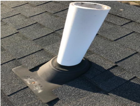
Pipe collars are in good condition and only minor sealing is needed on exposed nail heads.
