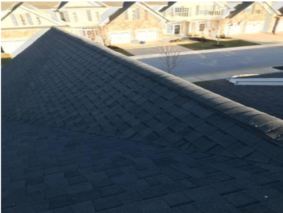
This picture shows over view of front elevation. Valley and Ridge vent appear to be in good condition
