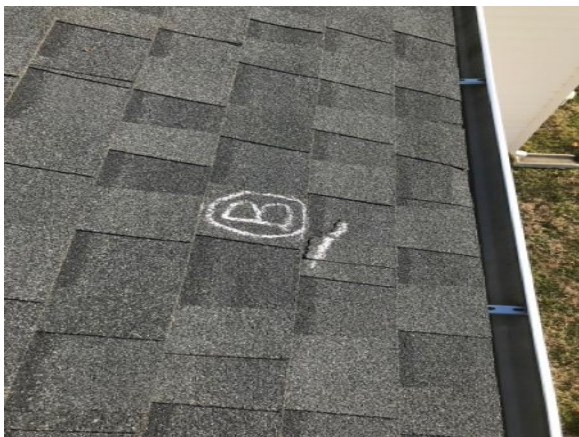
This picture shows damaged shingle on back elevation
