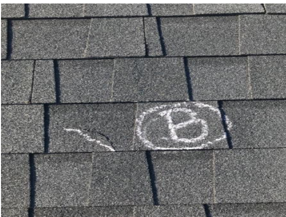
This picture shows cracked shingle on back elevation
