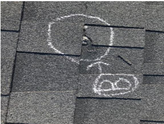
This picture shows nail pops and damaged on back elevation
