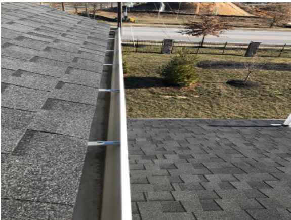
Gutters are clean and in good condition
