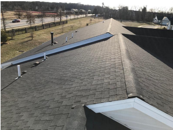
This picture shows ridge vent system on peaks of roofs
