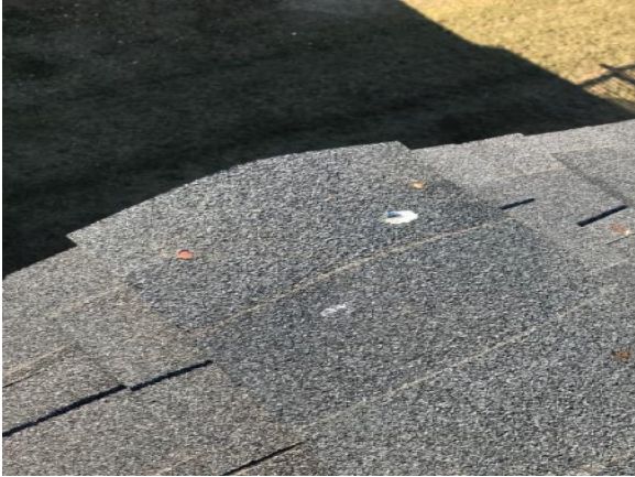
This picture shows ridge vent on back elevation and exposed nail heads on ridge
