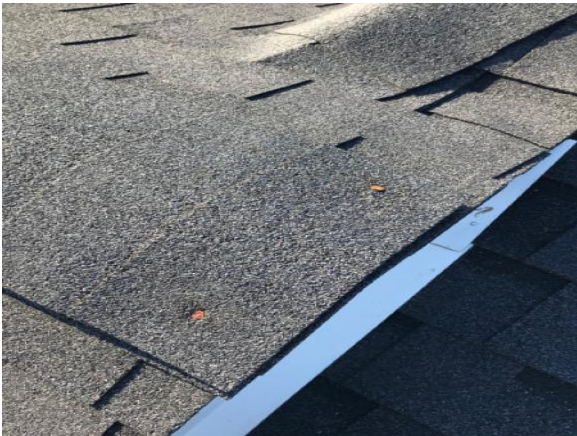
This picture shows ridge vent on back elevation and exposed nail heads on ridge. Sealant of exposed nail heads are recommended.
