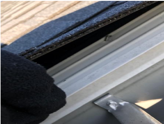
This picture shows drip edge is installed on this roof and appears to be in good condition
