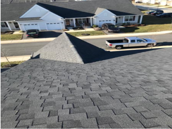
This picture shows over view of front elevation. Valleys and ridge vents appear to be in good condition.
