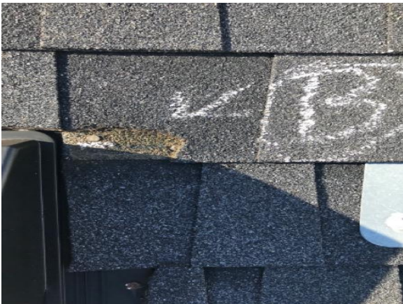
This picture shows damaged shingle on back elevation around bathroom/dryer vent
