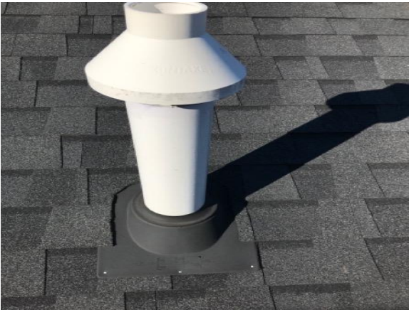
Pipe collars appear to be in good condition
