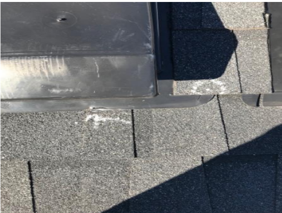
This picture shows exposed nail heads around dryer vents.
