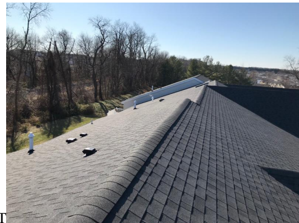
This picture shows over view of middle of building and ridge vent system
