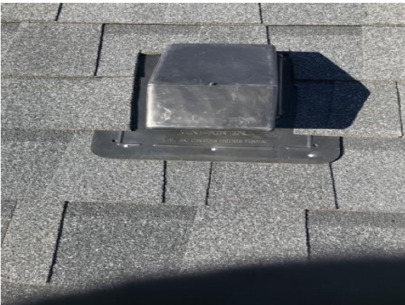
This picture shows some exposed nail heads on bathroom/dryer vents. Sealing is recommended and dryer vent cleaning is recommended
