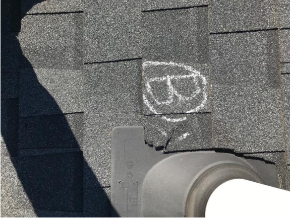
This picture shows damaged shingle around pipe collar on back elevation
